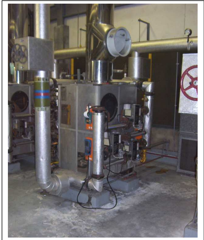
Ideal Concord, Super 50-300VH Model 200 231kWh input rating 40mm external dia steel supply pipe
